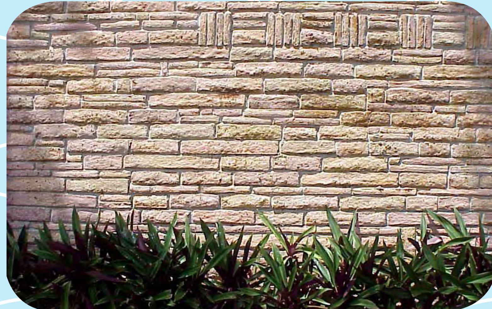
Brick and slumped brick
